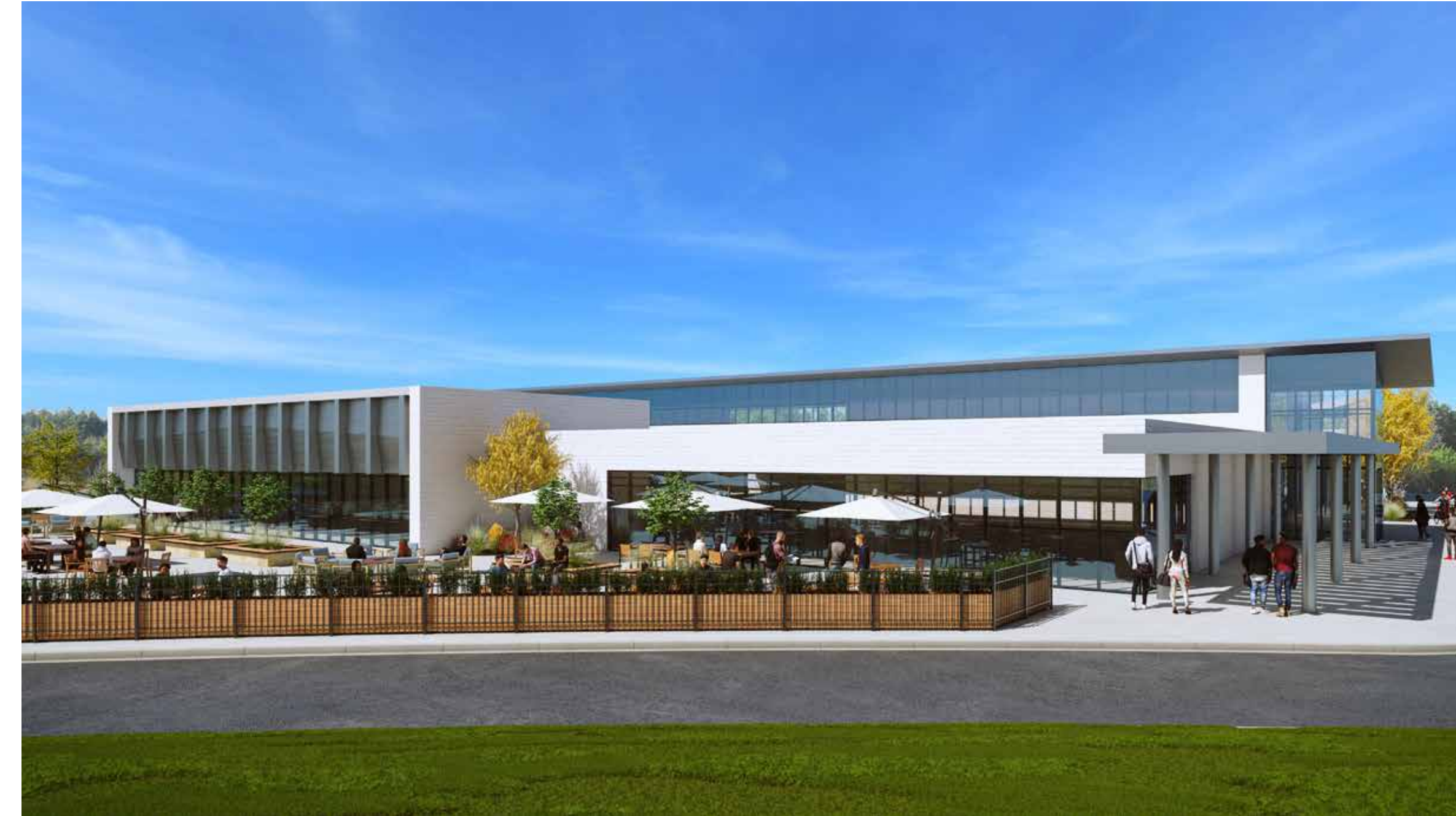
The Duncan Building exterior North Facade from the Valley Children's Stadium. The outdoor space north of the training table will transition from gameday club environment to an outdoor plaza and multi-use event space for all athletic teams.
