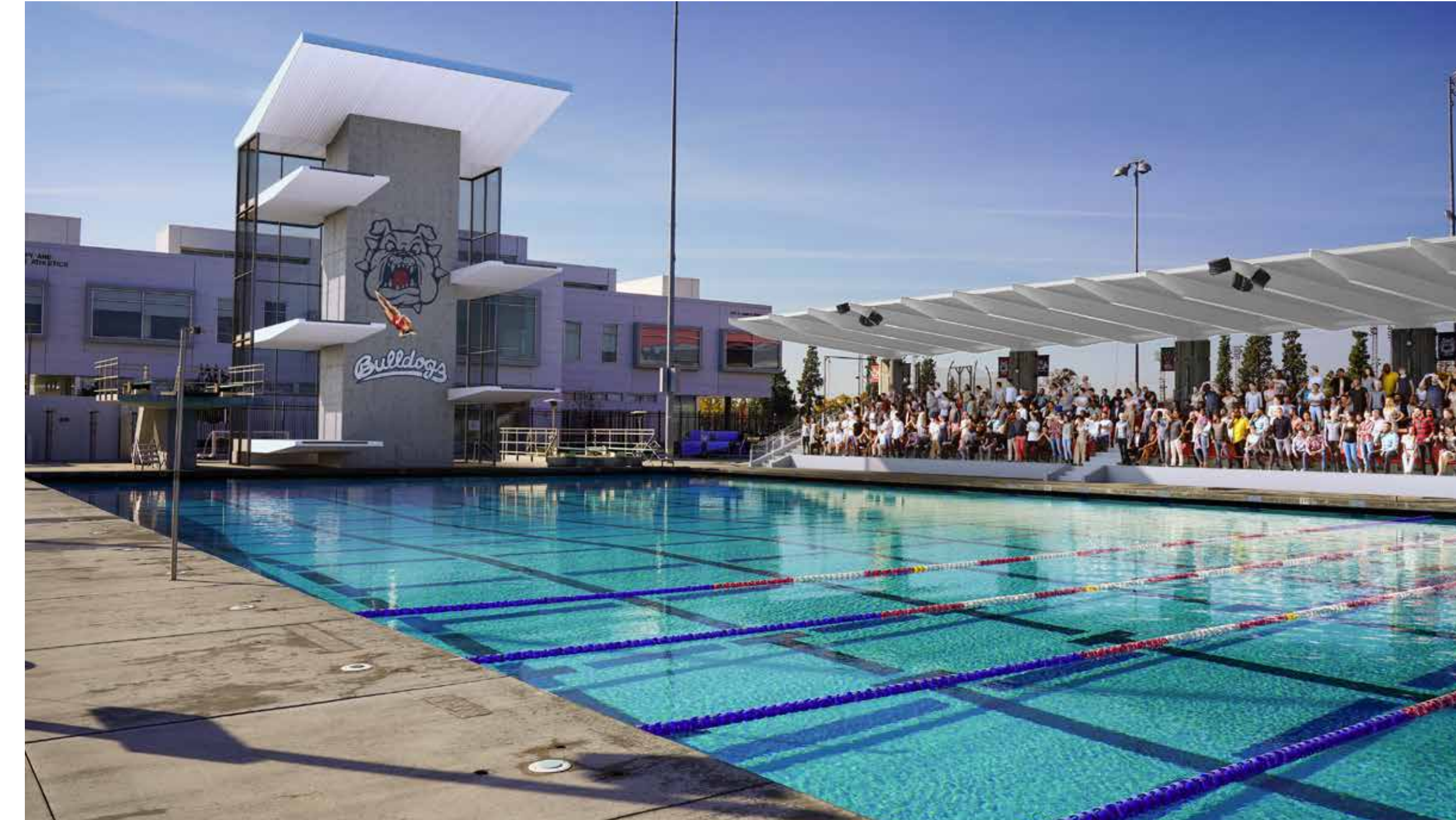
The new dive tower will be located on the south end of the aquatics center. The 10M dive tower will be the marquee feature of the aquatics center, an eye-catching image against the sky. The dive tower will attract top tier talent as well as allow the center to host multiple events and competitions. There will also be an enhancements to the aquatics spectator seating pavilion, and the locker rooms. In addition to adding the dive tower there will be a new aquatics center video board.
